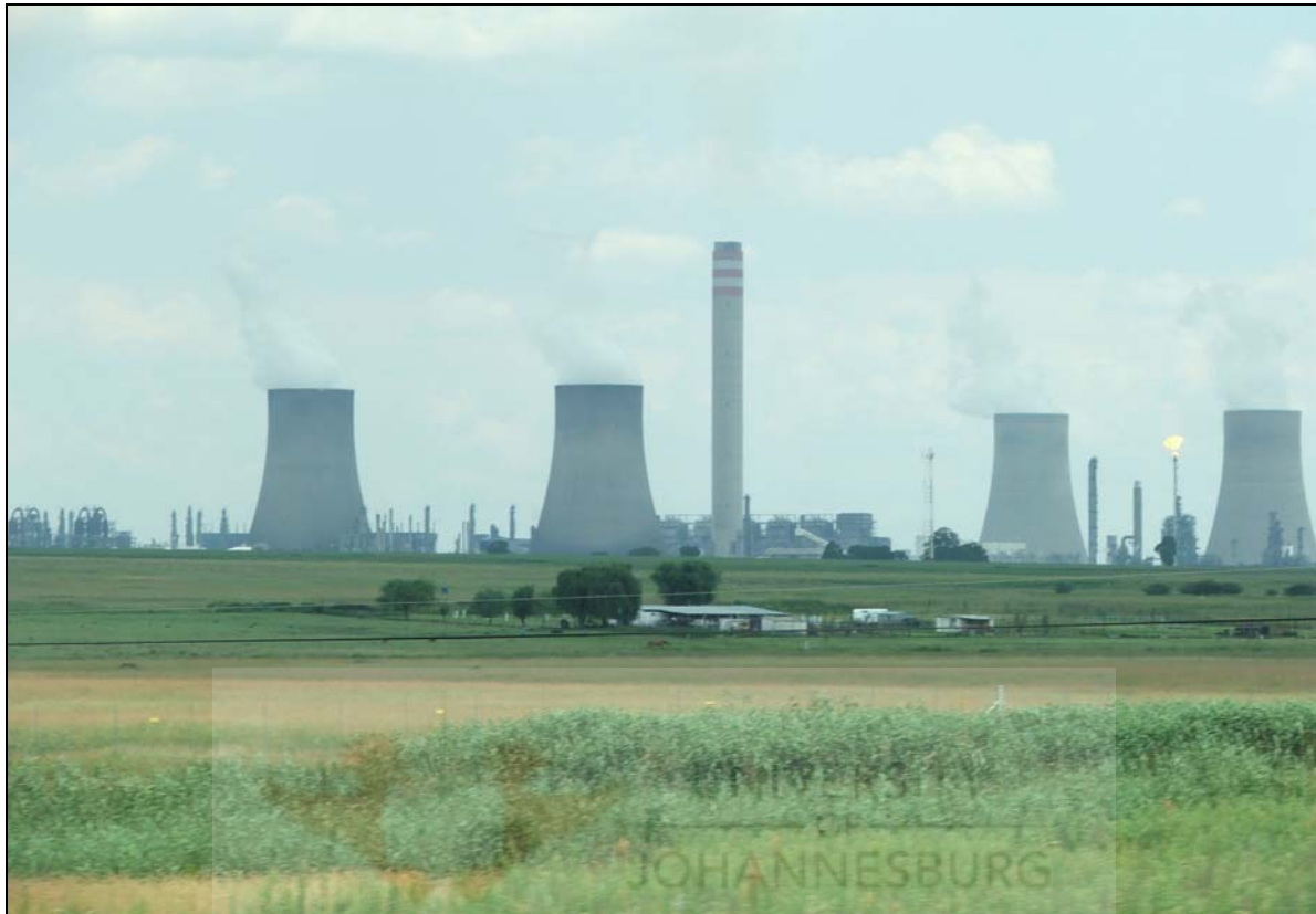
Figure 10: The Sasol Secunda Industrial Plant in Secunda, Mpumalanga.
