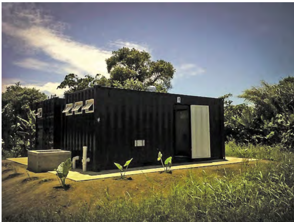
Figure 1 A typical CAB in Frasers informal settlement (Crous, 2012)
