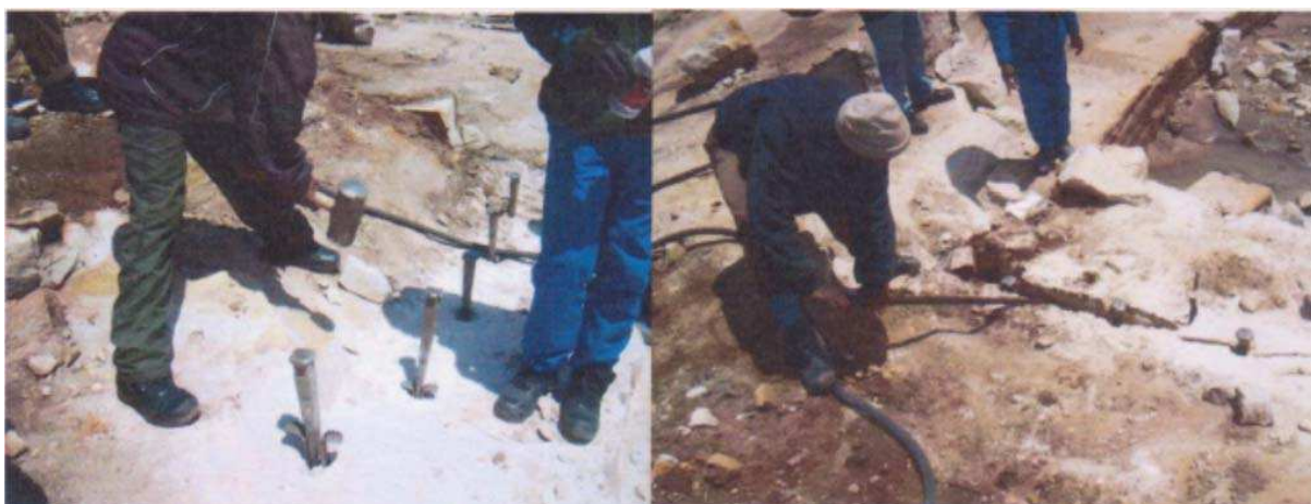
Figure 3: Rock breaking using Hammers and chisels in QwaQwa. Source: Tshabalala [15].
