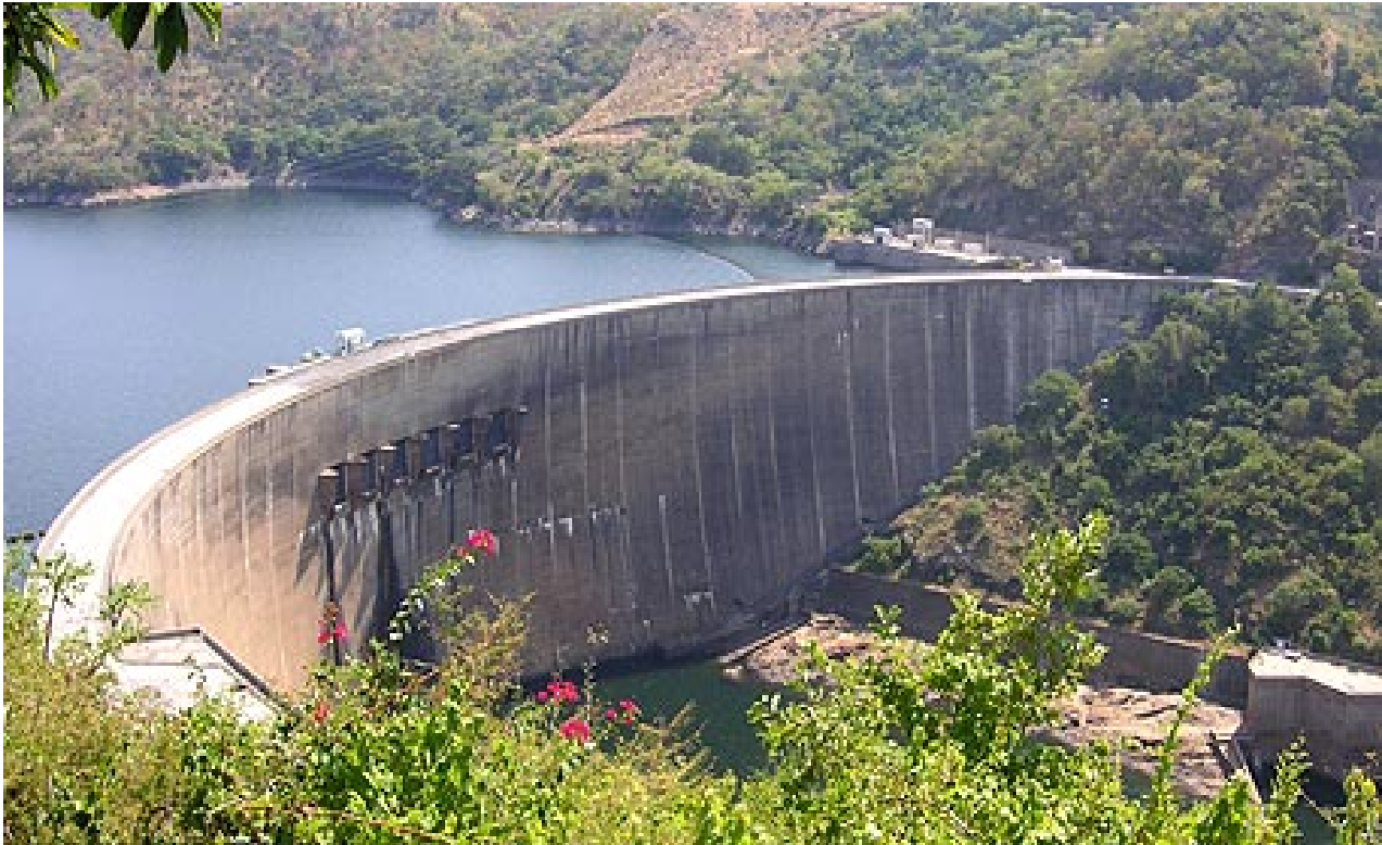
Fig1: Kariba concrete arch dam
