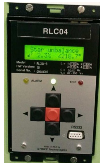
Figure 5: Current unbalance level on commissioning
