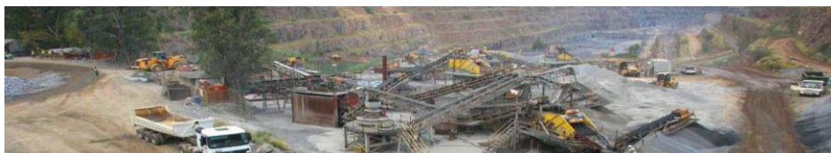
Figure 1. Lyttelton dolomite mine
