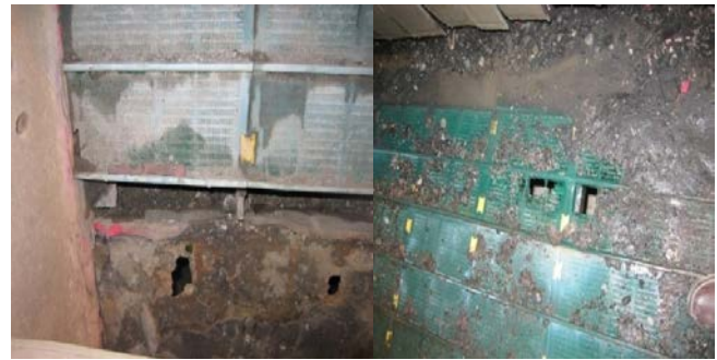
Fig. 7a: Holed screen panels and surface
