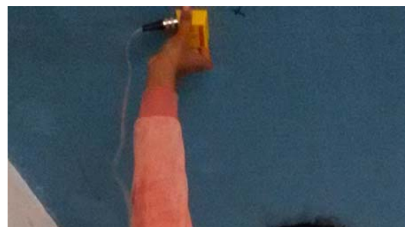
Fig. 5. Cover-meter measurement at the soffit of the roof slab.
