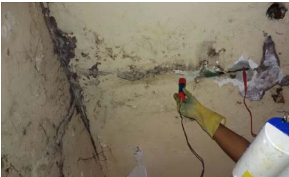
Fig. 7. Ongoing half-cell potential measurement at the soffit of the roof slab.
