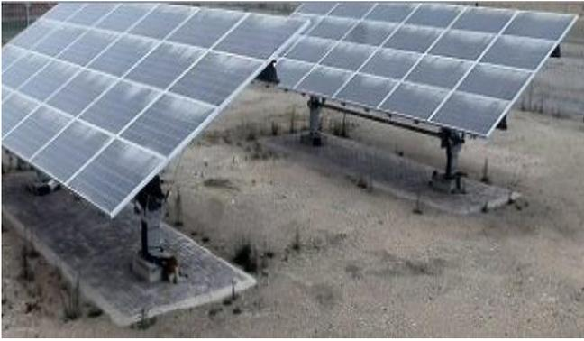
**Figure 2: Pilot PV system with single-axis solar tracking installed in Limpopo, South Africa**
