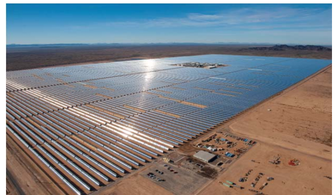
Fig. 3 Solana Generating Station in Gila Bend, Arizona, which is currently the world's largest parabolic trough plant [8]
