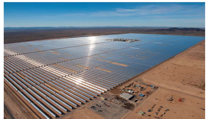
Fig. 3 Solana Generating Station in Gila Bend, Arizona, which is currently the world's largest parabolic trough plant [8]
