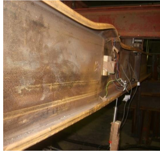
(b) Outward deflection of flange
