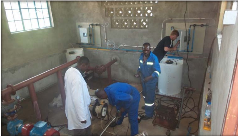
Figure 4. Technical Staff at Work Installing the Chlorinators in the Pump House
