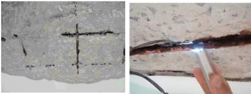
**Figure 1.** Effects of thin concrete cover on corrosion of steel reinforcement; (a) slab soffits (b) beam [5]
