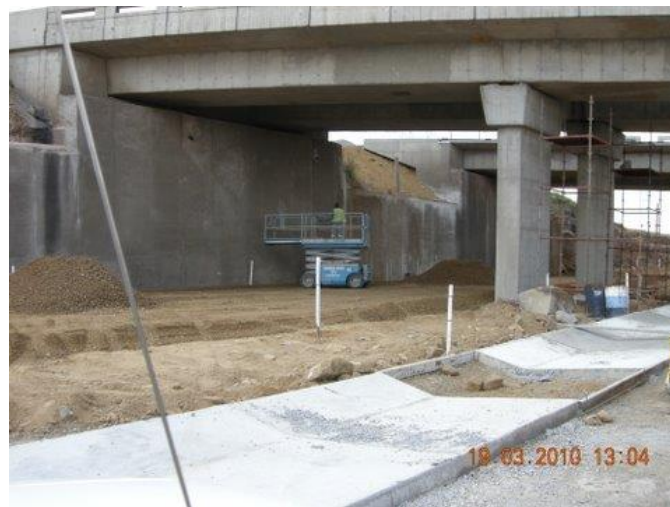
Figure 2. A newly completed highway bridge structure
