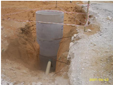
Fig 1: Manholes installed in deep excavations
