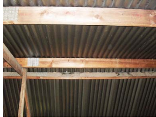
Figure 7: Source- Site Visit
