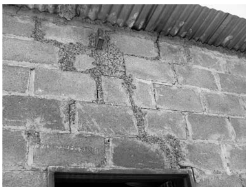
Figure 4: Source- Site Visit
