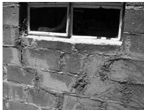
Figure 5: Source- Site Visit
