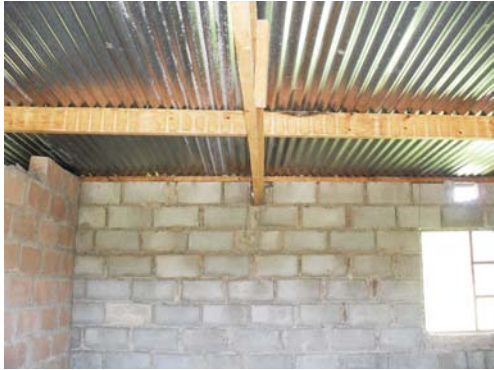
Figure 6: Source- Site Visit
