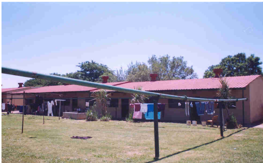
Photograph 6. The outside of Number 2 Hostel
