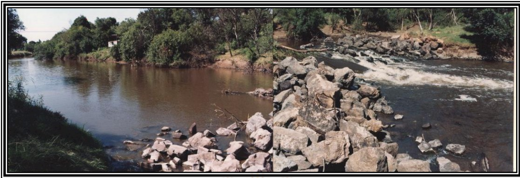
February 1998, upstream view.
