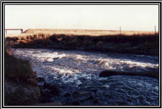
May 1998, downstream view. (note extensive bank erosion).
